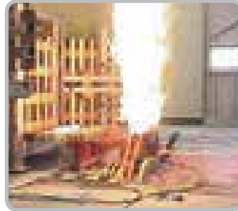
Short-Circuit Test / ACB Breaker Test
