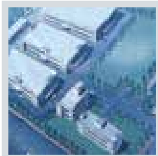
Wuxi Plant (China)
